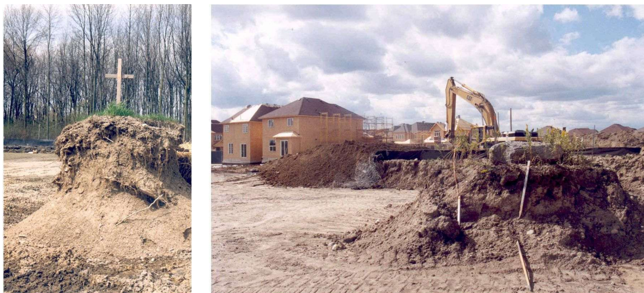
Figure 13. Soil is removed to standardize the relationship of houses to grade, speeding up construction and centralizing stormwater management.
