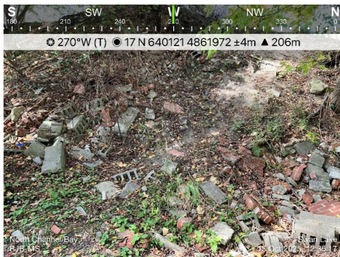
Photo 1: North Channel Dry at Time of Inspection, Containing Remnants of Landfill Waste. Represents a Beautification and Bioswale Opportunity
