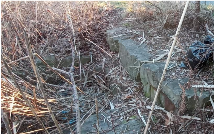
East Pond Mid-Splitter Before Cleaning (Dec 2021)
