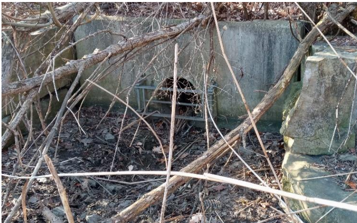
East Pond –Inlet from South Splitter (April 2022)
