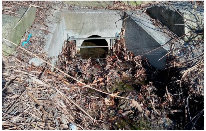
East Pond Mid-Splitter After Cleaning (April 2022)
