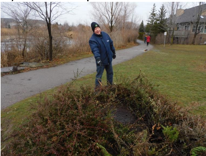
Buried Separator found in 2020. Possibly cleaned in fall of 2020.
