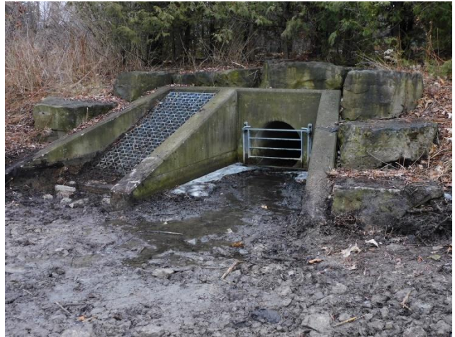
Lake Outlet December 2020 (After clearing)
