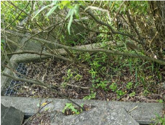
Lake Outlet June 25, 2020 (Before clearing) 5
