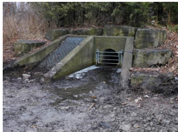
Lake Outlet and South Inlet Pipe December 2020 (After clearing)
